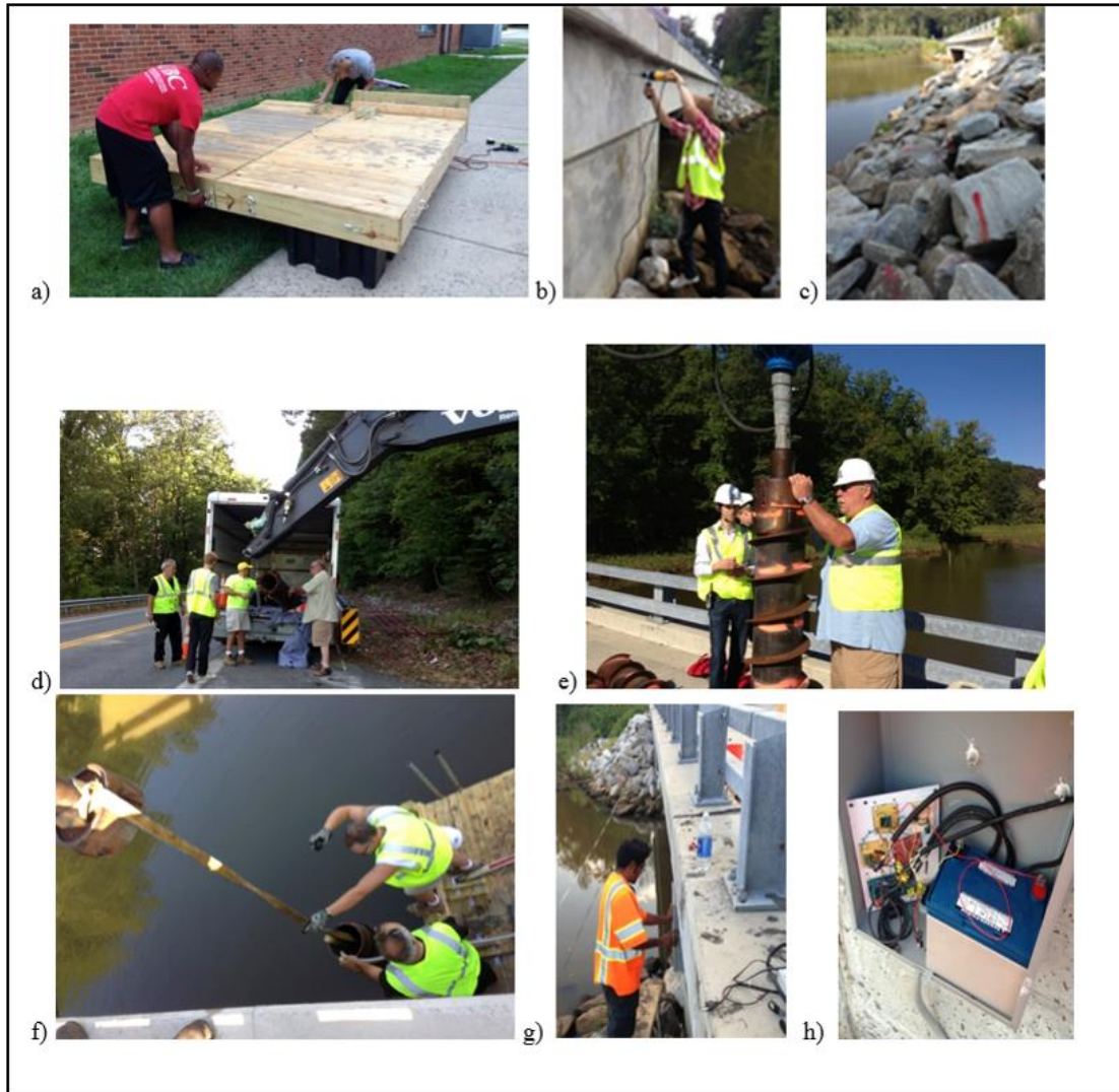
Figure 35. Photos of full-scale installation at Bridge No. 02072 on MD450 over Bacon Ridge Branch. a) students building installation working platform; b) installation of electronics housing on bridge structure; c) contact Miss Utility well in advance
