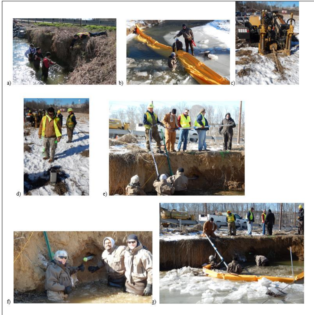
Figure 46. Photos of full-scale installation at Bridge No. 1008600 on MD355 over Bennett Creek. a) Jeff Knaub of MDSHA showing UMD students target location for sensors; Rip rap protecting bank from prior scour event at top left of photo; b) installation of turbidity curtain on morning of installation; c) BelAir drill rig ~9.2m (30 ft) from where sensor will protrude from bank; d) sensor used to track depth and lateral position of drill tip; e) feeding wiring and sensor post into bank ~60 cm (2 ft) above nominal water level as drill bit is retracted; f) admiring successful installation of the in-air sensor post; g) feeding wiring and sensor post into bank at depth of ~15.25cm (6 inches) below nominal water level for this site.
